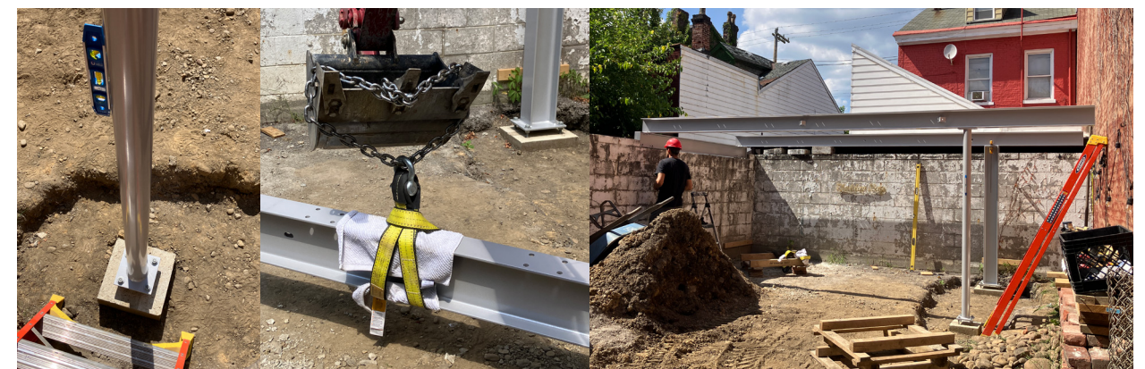
(Top) Excerpts from structural steel shop drawings for fabrication. (Bottom) Construction photos of steel receiving and erection.
