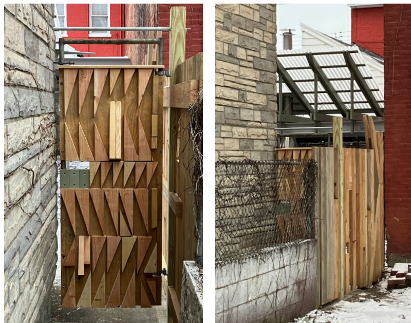
(Bottom) New access gate and privacy fence made from salvaged steel gate frame, wood truss prototype, and assorted project offcuts. (Opposite) Detail of horizontal steel tie rods and underside of galvanized steel valley gutter.
