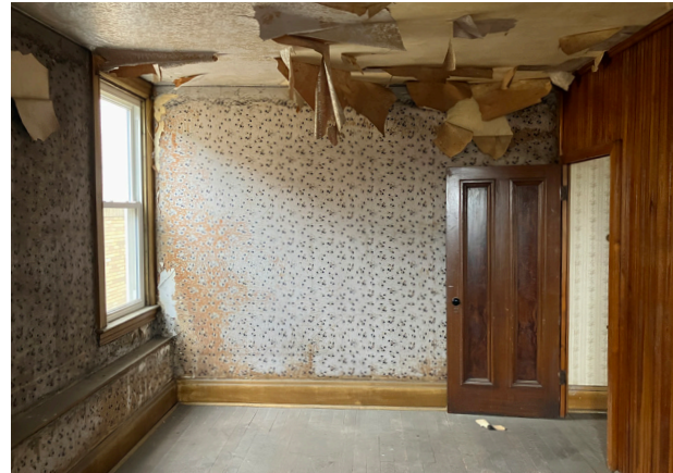
Third Floor: existing north bedroom
