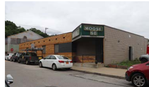
Exterior photograph of the Millvale Moose building.
