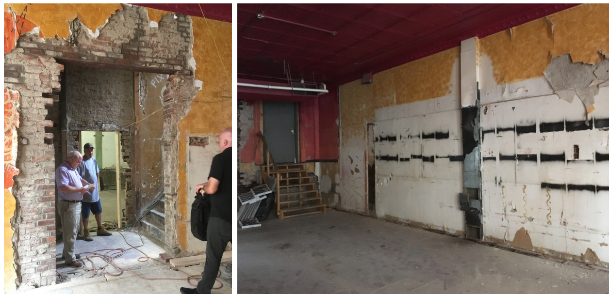
Photographs of existing structure before and during selective deconstruction.
