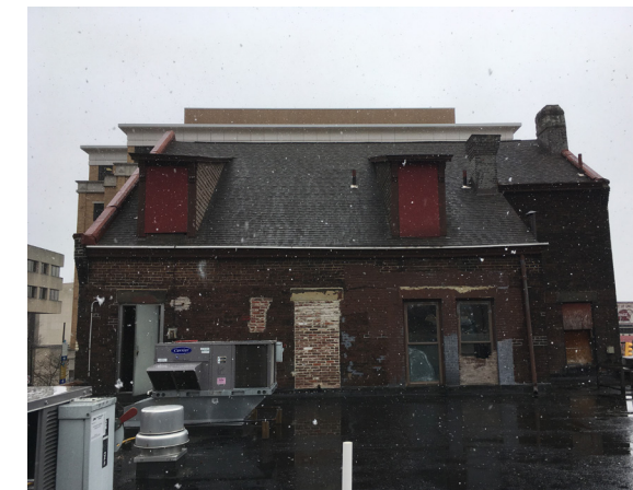
Original north facade and roof.
