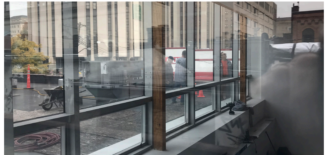
Photographs of nearly completed building. All new interior surfaces were left pure and white, celebrating the textures and tones of existing masonry, new LVL structural members, and view out the new north-facing curtain wall. (Photos by John Folan)
