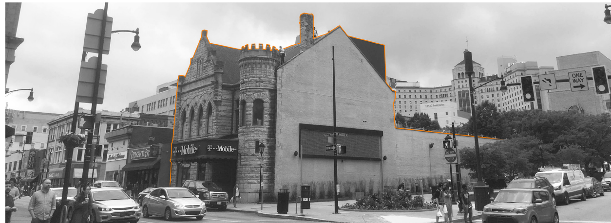
(Above) Photograph of King's Court building from across Forbes Avenue, northeastern corner of new addition visible in rear; (Opposite) Photograph of new north-facing curtain wall emerging from the roof of the existing building.
